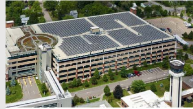
Utility-scale solar array on the BTV parking garage
