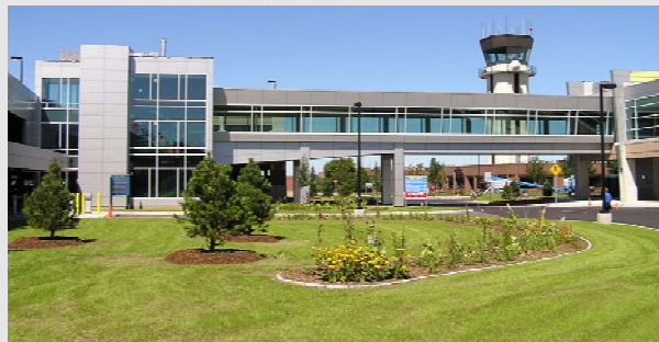
Pedestrian Bridge from the Parking Garage at BTV
