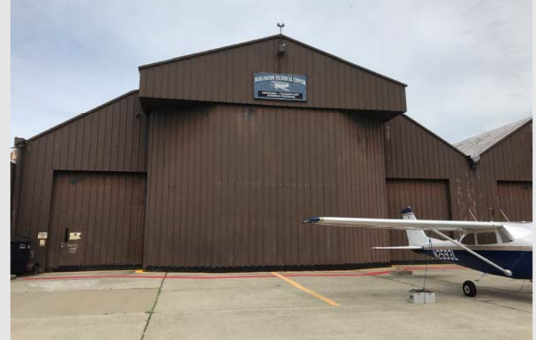
Alert Hangar at BTV Credit: VHB
