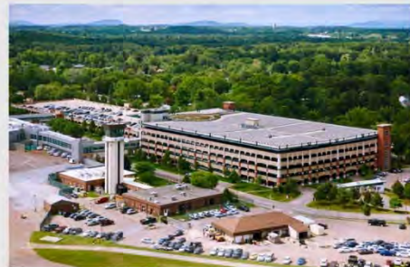
Solar Photovoltaic System at BTV Credit: Vermont ANG
