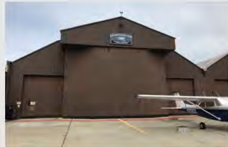
Alert Hangar at BTV Credit: VHB
